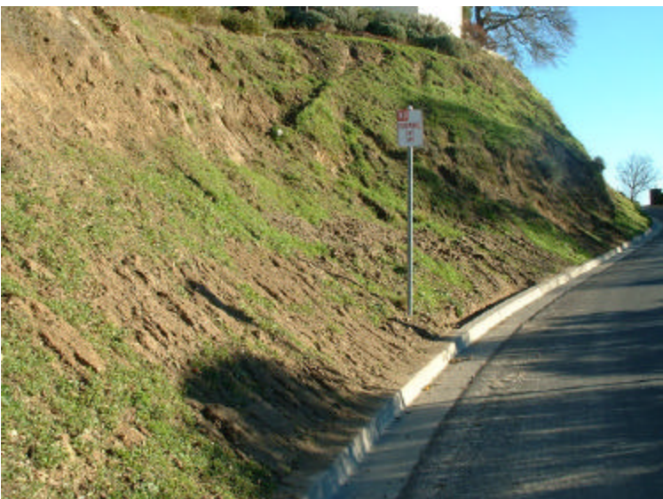
Figure 8. Eroded soil from above is spilling over curb and onto roadway. Almost no vegetation roots are remaining to keep soil from further erosion.
