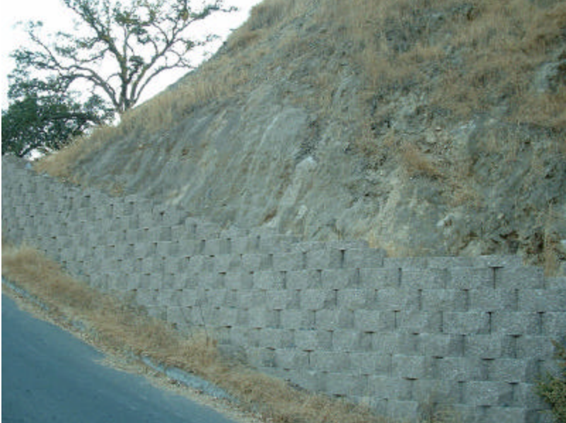
Figure 2. Interlocking retaining wall blocks without plantings.
