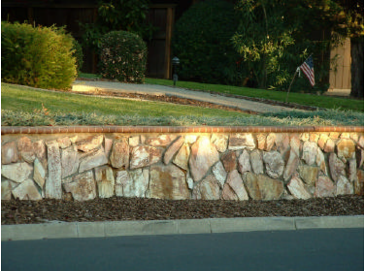
Figure 3. A “first-class” retaining wall.
